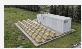
A key milestone for the RHE-MEDiation project: the **GreenDune® photobioreactor**, developed by BLUEMATER SA, **has been installed in Türkiye**. The system will treat primary-treated wastewater—rich in nutrients but high in suspended solids—using microalgae.
